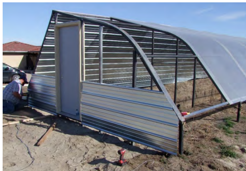
Construction of Finch's passive solar greenhouse. Photo: Russ Finch
