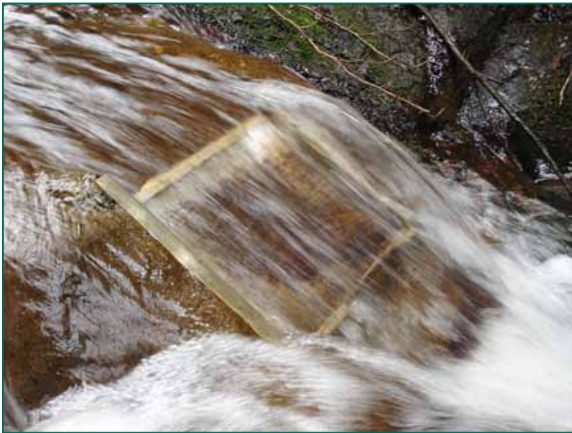
Intakes should be carefully located to take on characteristics of the natural stream flow. Photo: Leif Kindberg, NCAT
