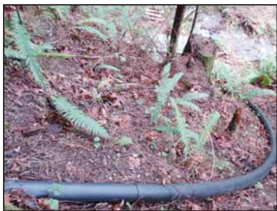
High-density polyethylene (HDPE) pipe is durable and manages bends better than rigid PVC or steel pipe. Photo: Leif Kindberg, NCAT
